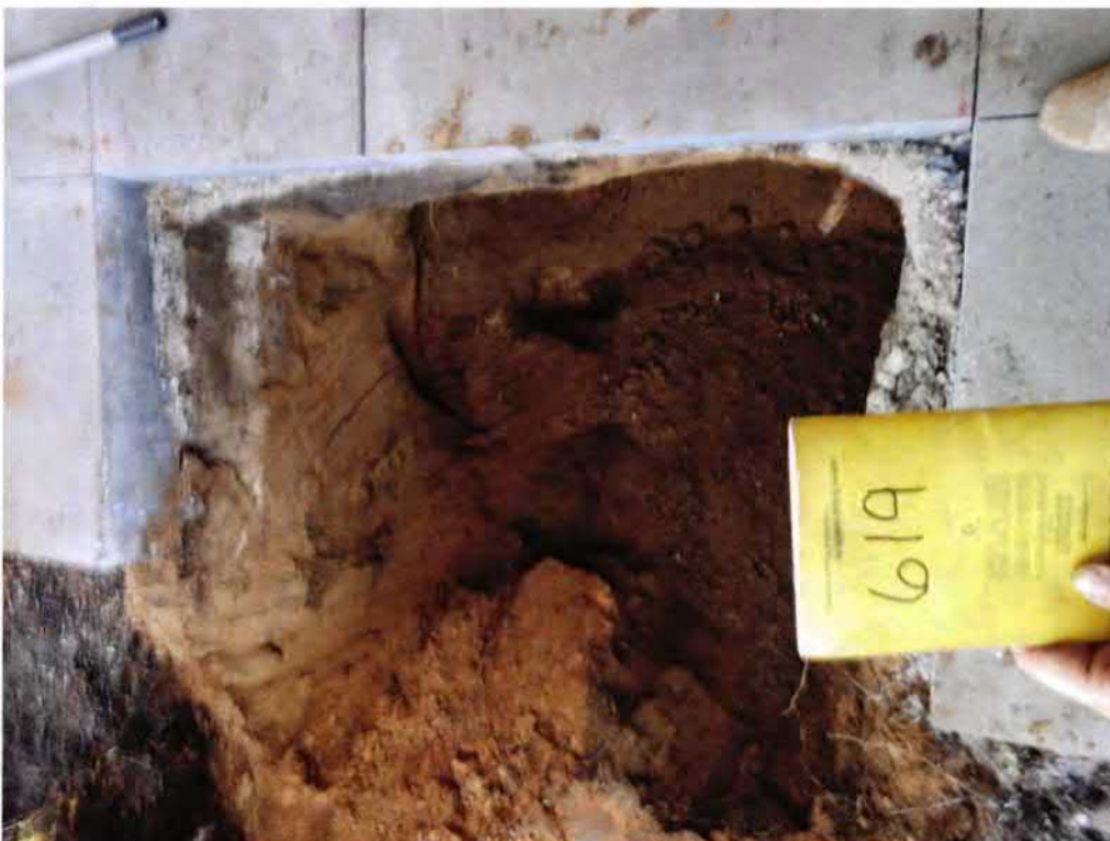
Picture 2: UST 619Dahlia excavation.
